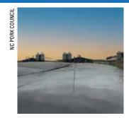
Capturing Methane on the Farm As pig manure breaks down, it produces methane gas. Instead of allowing methane to enter the atmosphere, it's captured in a covered anaerobic digester. An initial cleaning removes condensation and other impurities.
