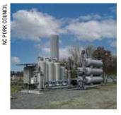
Converting Methane to RNG The methane captured from multiple farms is sent via low-pressure pipes to a central conditioning facility, where it's refined to 99% pure methane, the same as traditional natural gas. The gas goes through a two-step testing process before entering the natural gas pipeline.
